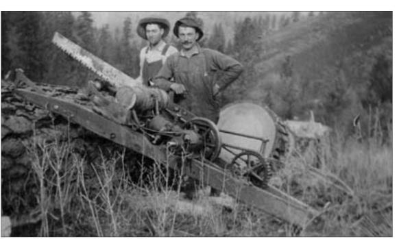
These Idaho County loggers are using a gas-powered cross-cut saw in this undated photo.
